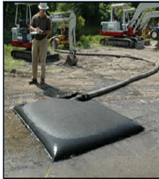
Plate 4-4. Silt Bag under inspection.
