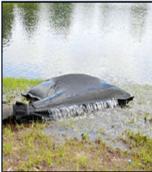
Plate 4-3. Silt Bag with water being pumped through.
