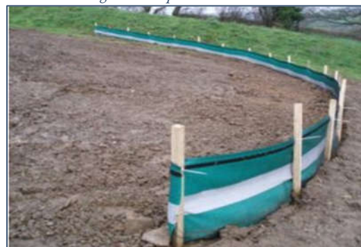
Plate 4-6. Embedded Silt Fence
